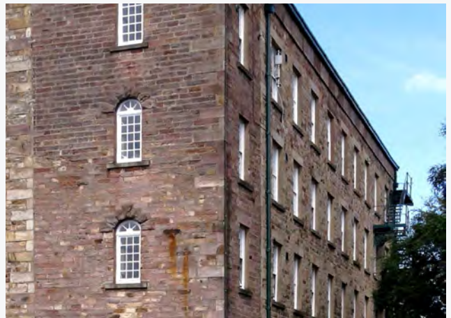
Moor Lane Mills scheme (Source: Alan Marsh)
