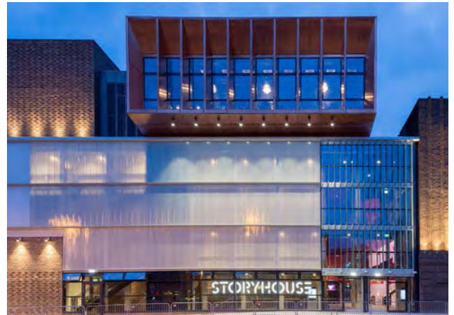
Figure 57 Storyhouse, Chester (Source: Bennetts Associates)
