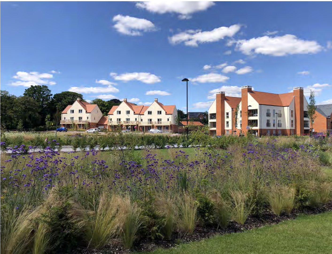
Figure 33 Barton Farm development to north west of Winchester (Source: JTP)
