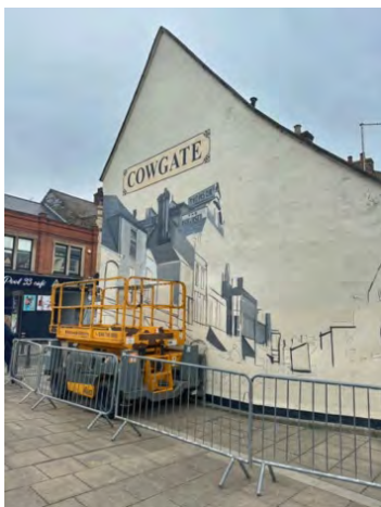
Cowgate mural under construction, 28 February 2024
